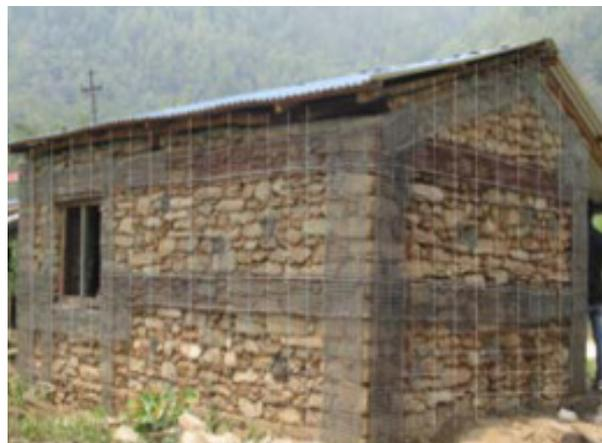
Figure 3: Containment Reinforcement (CR) system
