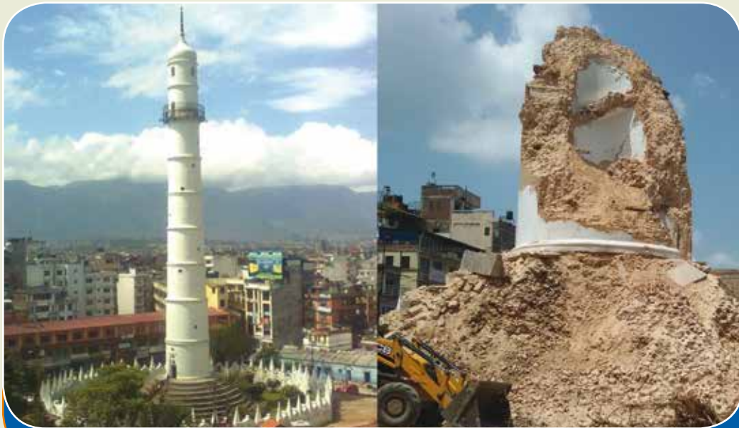
Photo: Dharahara (Icon of Kathmandu)—before & after the earthquake
