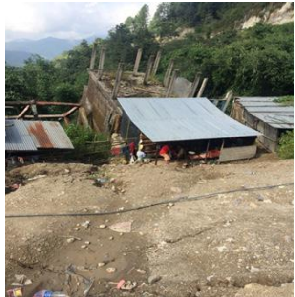
Pic 3: Houses at risk from the Kapurkot Landslide Pic: Survey Team
