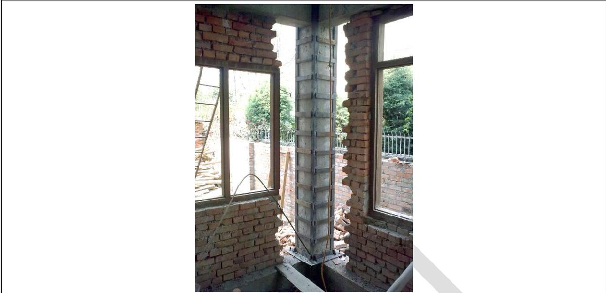
*Fig11: Retrofitting of columns by steel profile jacketing*
