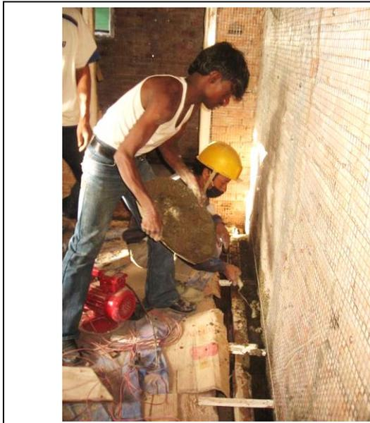
*Fig 5: GI wire mesh jacketing*
