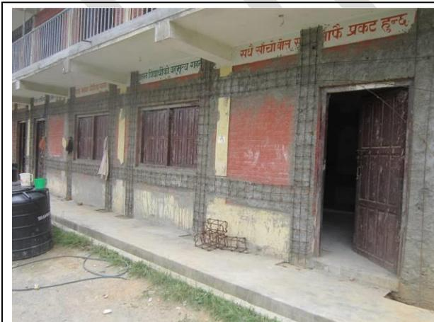
*Fig13: Strengthening of infill masonry wall of RC frame building through RC Splint and Bandage method*
