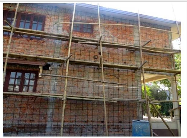
*Fig 14: Strengthening of infill masonry wall of RC frame building through RC jacketing method*
