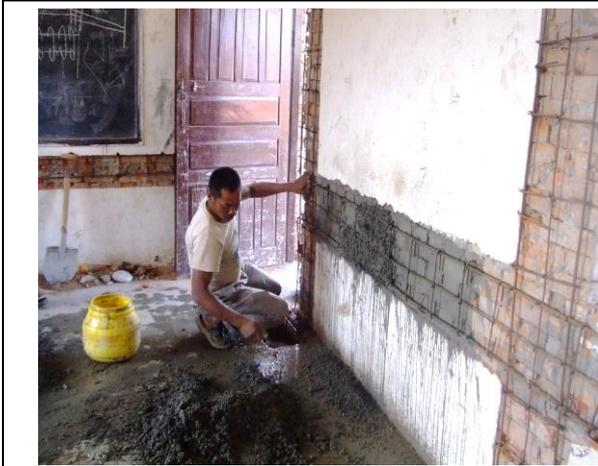
Fig 2: Construction of RC splint and Bandage
