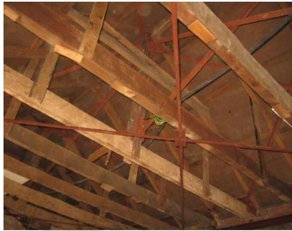
*Fig 17: Addition of bracings to flexible floors*
