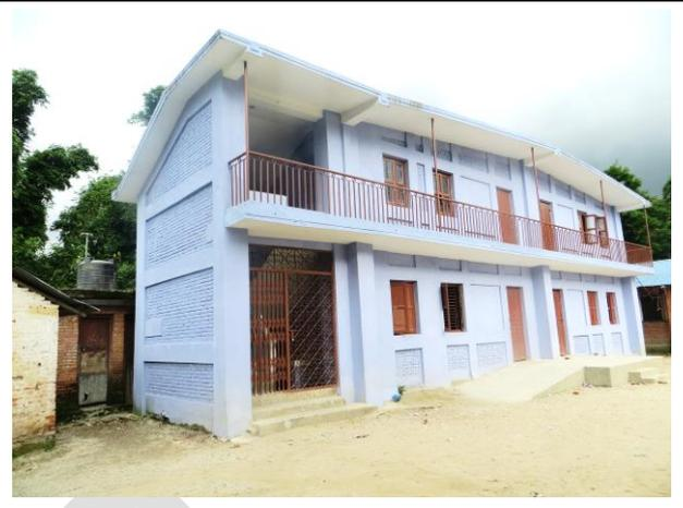
Fig 3: Building retrofitted by RC splint and Bandage method
