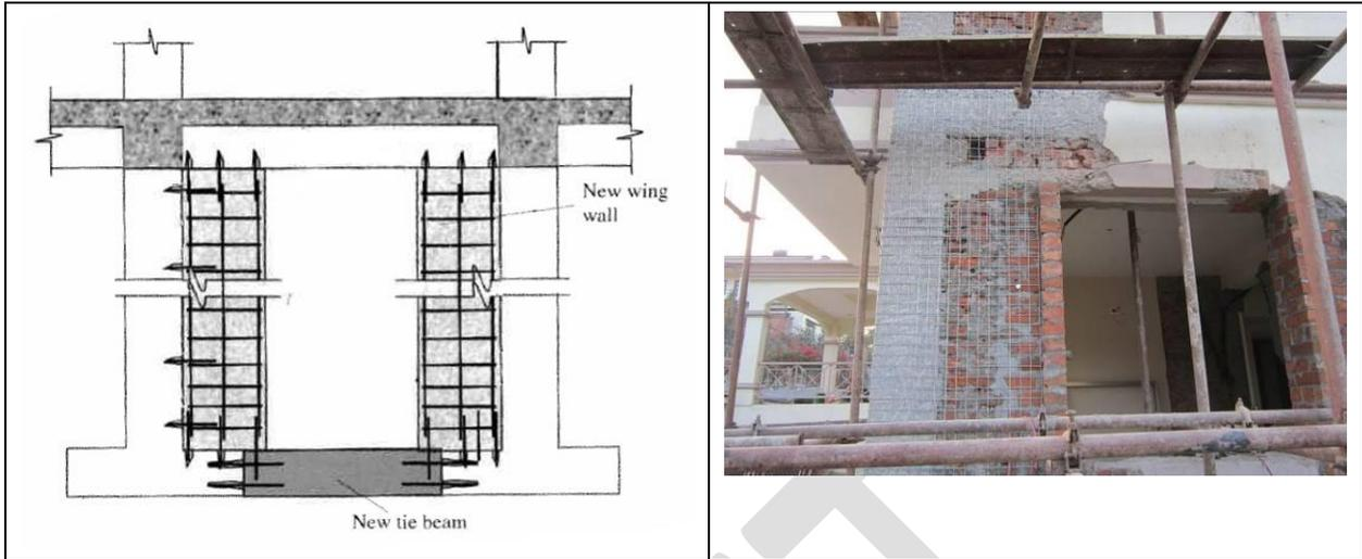
*Fig12: Strengthening of wing wall in RC Frame Building*
