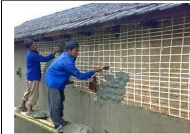
*Fig 7: Retrofitting using PP band*
