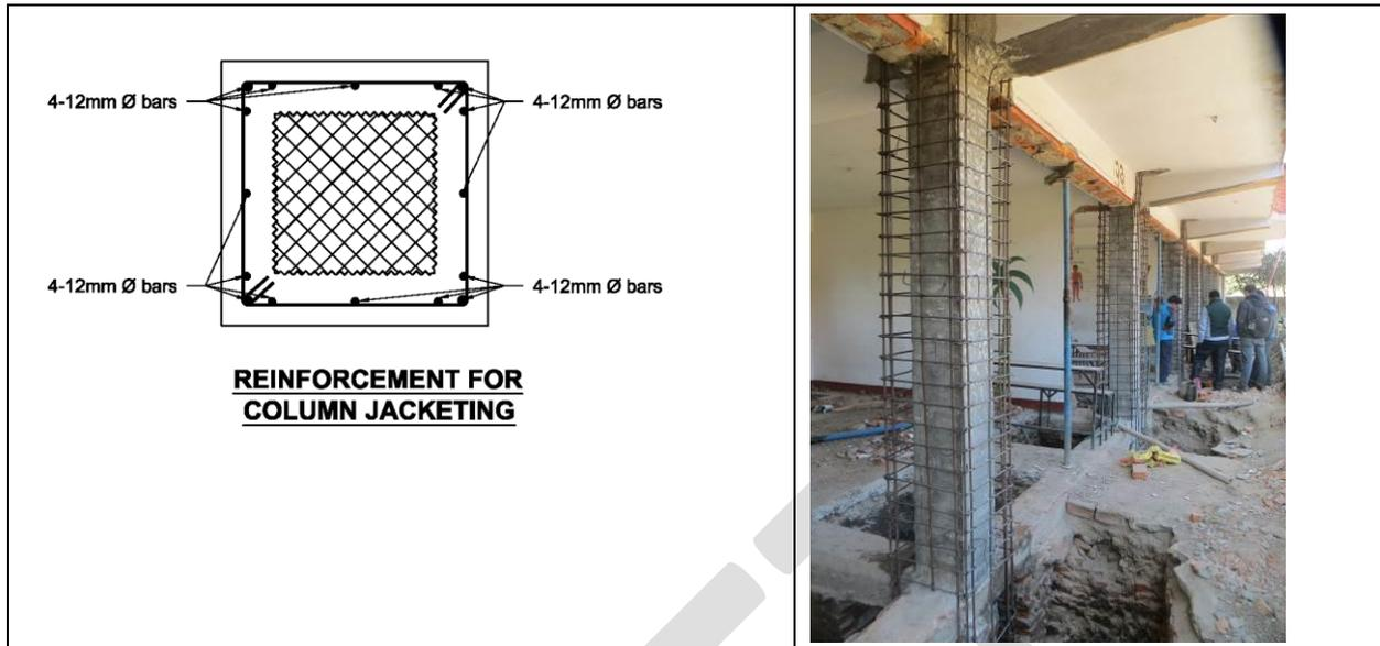
*Fig 9: Retrofitting of columns by RC jacketing*
