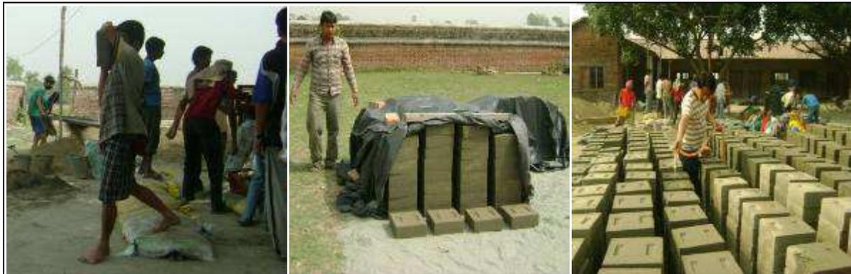
Figure 14 Carrying, storing and water curing of CSEB
