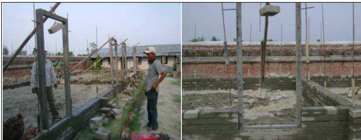
Figure 24 installation of door at plinth level
