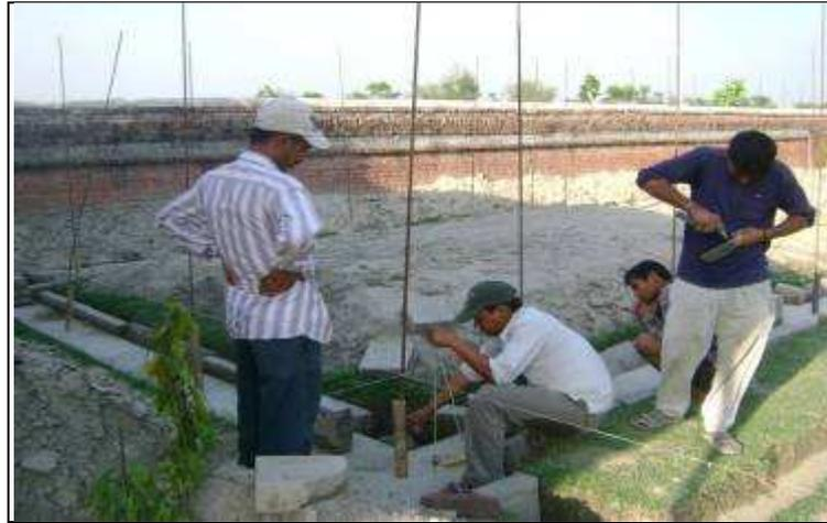
Figure 20 Completion of foundation ring beam
