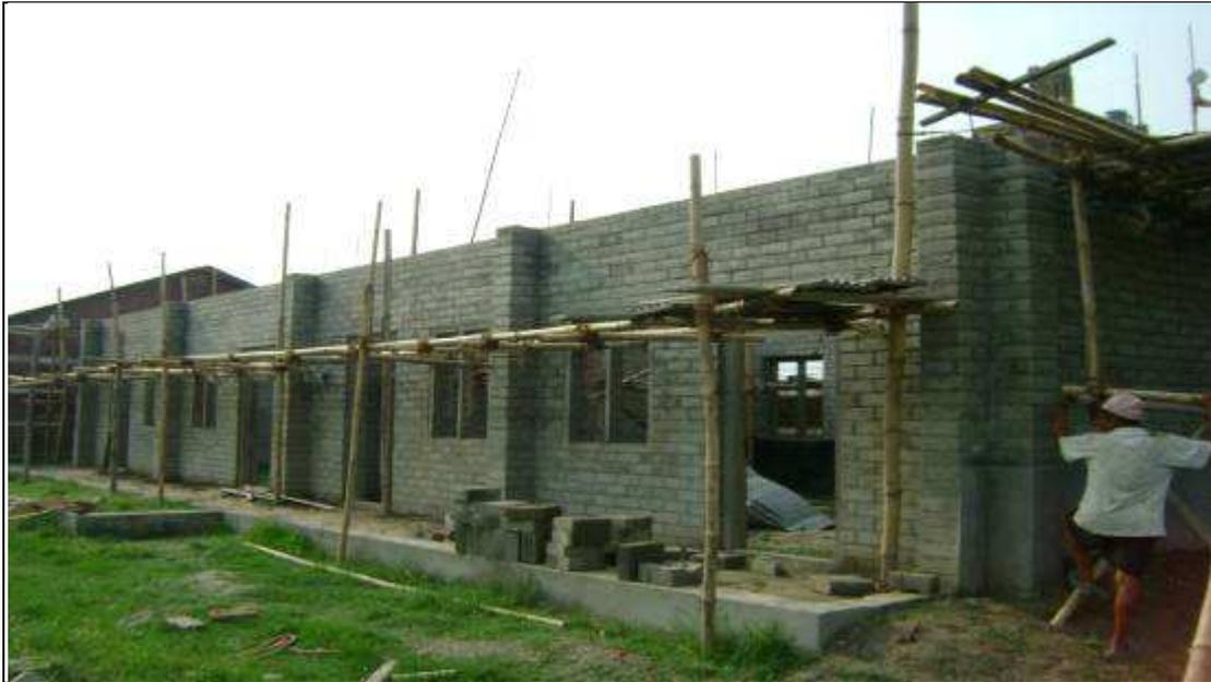
Figure 29 completion of lintel ring beam
