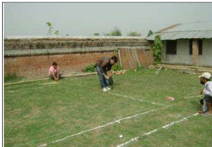
Figure 15 layout for excavation of foundation at Morang district
