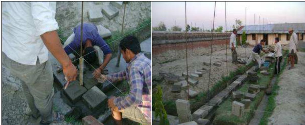
Figure 21 Starting of block work at first layer
