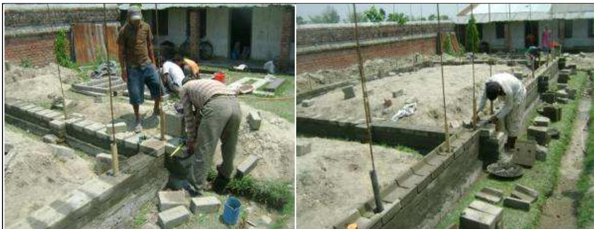
Figure 22 Block work at second layer and laying of U-block for plinth ring beam
