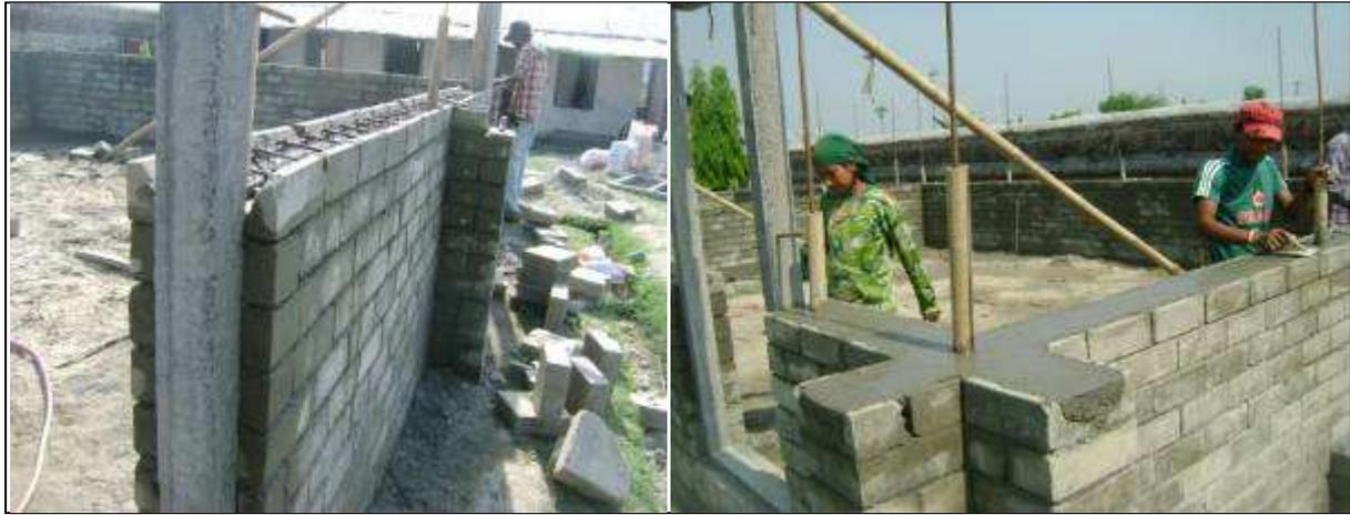
Figure 26 arrangement of reinforcement and concreting of sill ring beam
