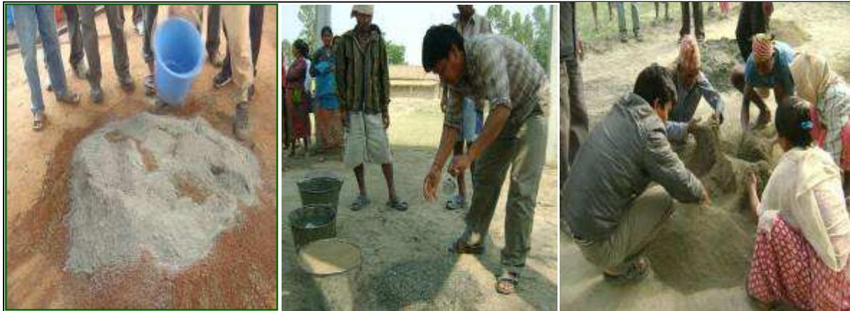
Figure 12 soil and cement mixing, sand and water mixing, and together mixing at Morang district
