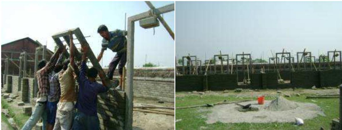
Figure 27 installation of windows above the sill ring beam
