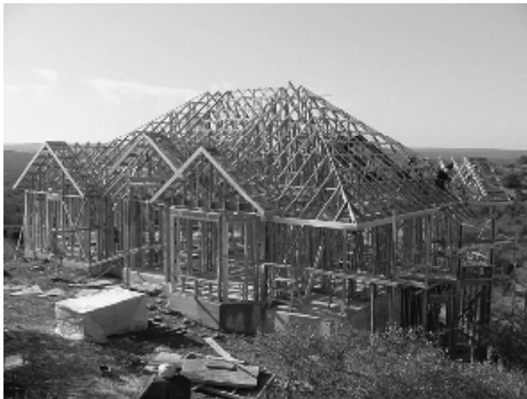
**Figure 5-13 Cold-formed steel house under construction.**
