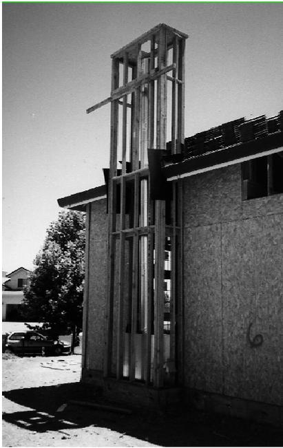
**Figure 7-7** Factory-built flue and light-frame enclosure.
