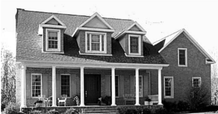
**Figure 5-14 House constructed with masonry walls.**
