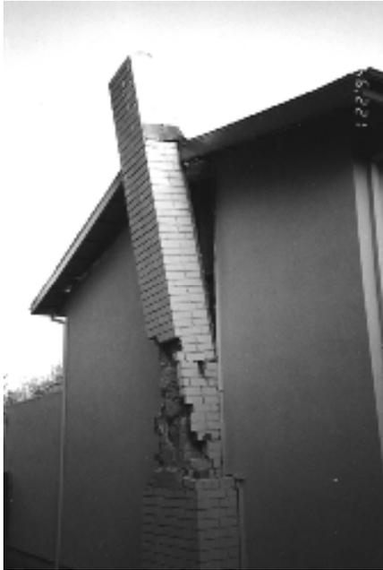
**Figure 7-2 Chimney damage in Northridge earthquake.**
