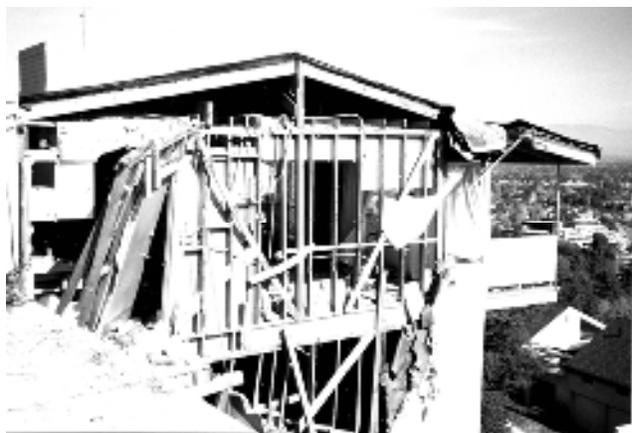
**Figure 9-10** House located on a hillside site damaged during the Northridge, California, earthquake.
