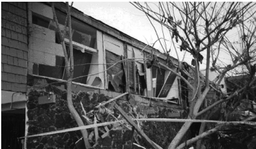
**Figure 5-12 Stone veneer damaged during the earthquake in Northridge, California.**
