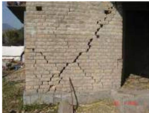
Photo 9: Diagonal cracking of solid wall (Bed joint sliding mode)
