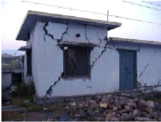
Photo7: Diagonal cracking of masonry piers starting from corner of openings
