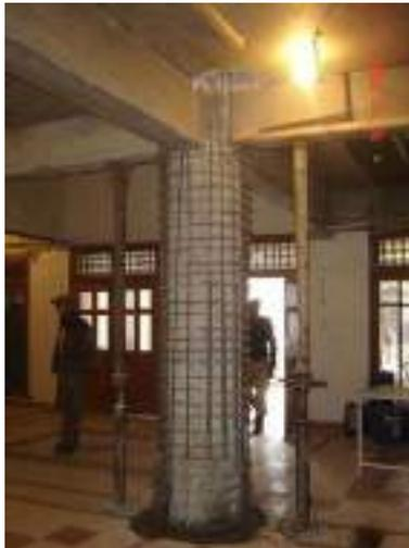
**Fig 10. (a) Jacketing of RC Column**
