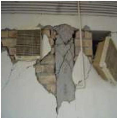
Photo 21: Shear crack in column
