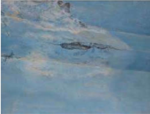
**Fig 2.9 (a) Delamination due to Seepage of Water**
