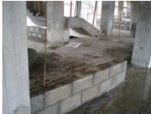
**Fig 2.12 (b) Tying of Infill Wall with Frame**
