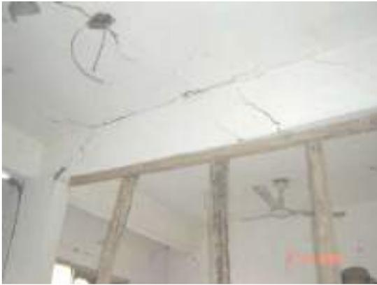
Photo 19: Shear cracks in beam near to support and at mid span
