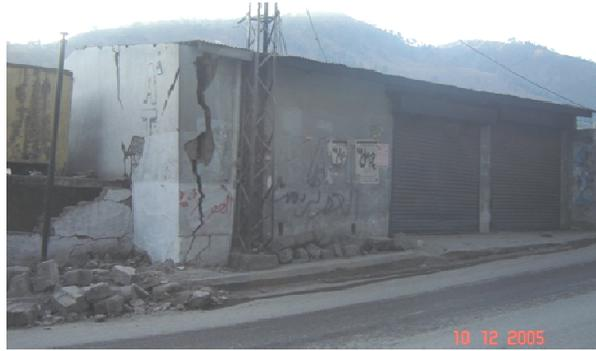
Large and extensive cracks in most walls, roof tiles detach, tilting or falling of chimneys, failure of individual non-structural elements such as partition/ gable walls. Load carrying capacity of structure is partially reduced.
