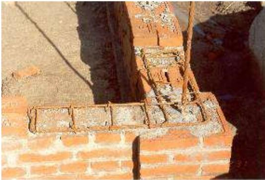
**Fig 2.16 (a) Vertical Reinforcement and Corner Stitch**
