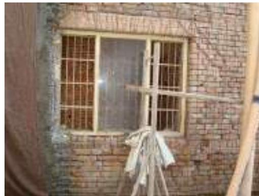
**Fig 5. (c) Wall Jacketing in Process**
