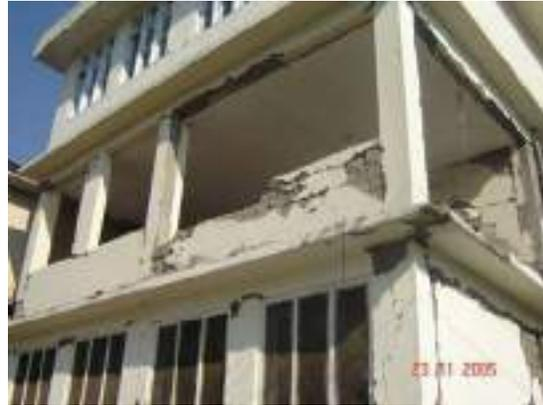
Photo 24: Extreme Damage to Infill wall
