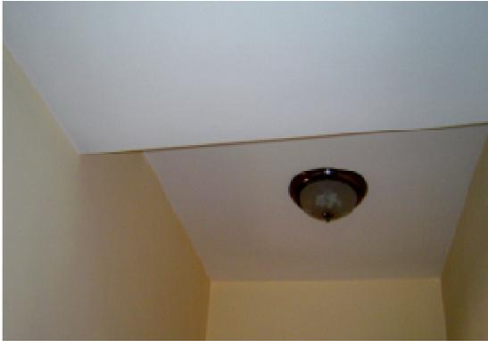
**Fig 2.17 (a) Drop in Floor Slab**
