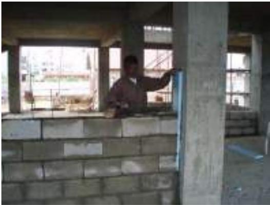
**Fig 2.12 (a) Separation of Infill Wall from Frame using Flexible Material**
