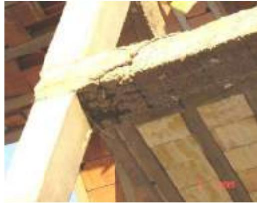
Photo 20: Shear crack in beam near to support
