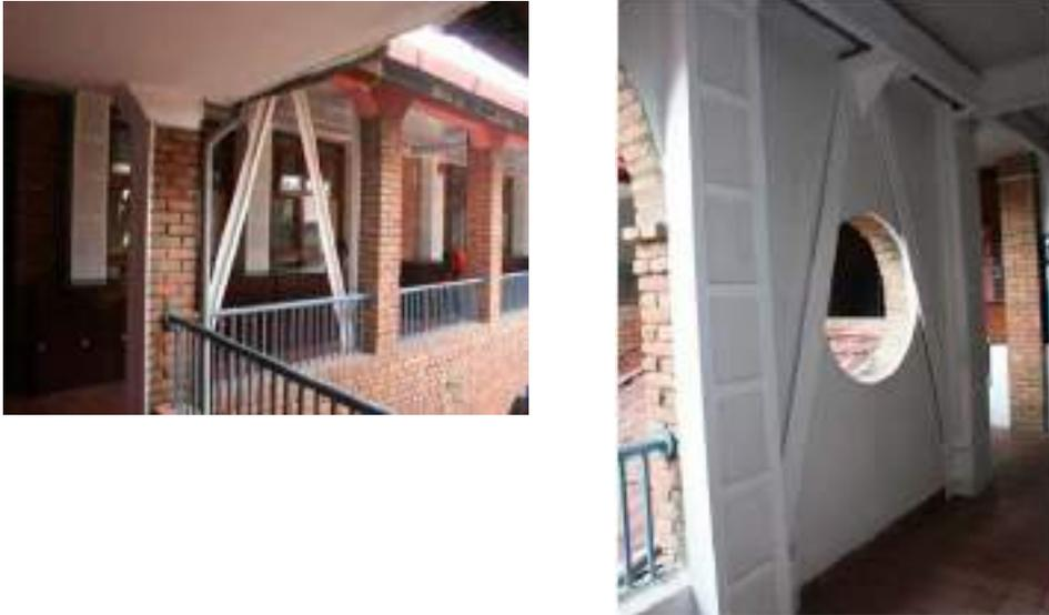
**Fig. 11. Retrofitting by Diagonal Steel Bracing**
