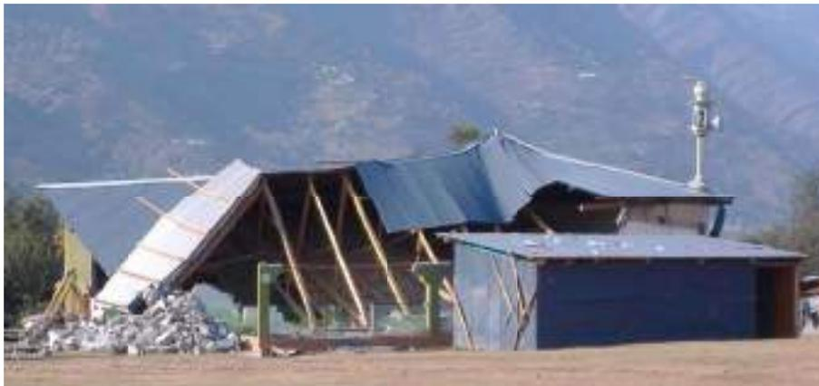
Gaps occur in walls, walls collapse, partial structural failure of floor/ roof, Building takes a dangers state.
