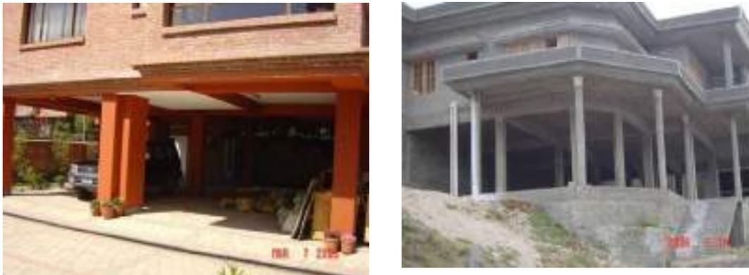
**Fig 2.5 (c) Soft Storey Problem due to Lack of Brick Infill in Ground Floor**
