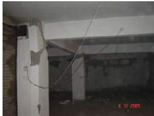
Large cracks in structural elements with compression failure of concrete and fracture of rebars, bond failure of beam bars, tilting of columns, collapse of few columns or single upper floor
