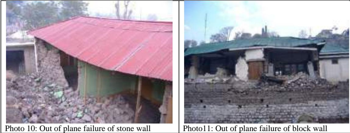
Photo 10: Out of plane failure of stone wall
