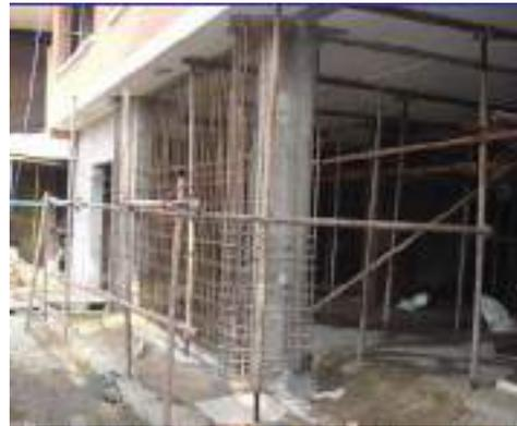
**Fig 10. (b) Addition of Shear Wall and Column Jacketing**
