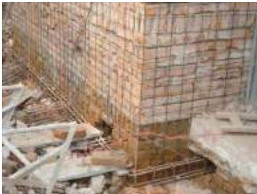
**Fig 5. (b) Erection of Reinforcement for Wall Jacketing**
