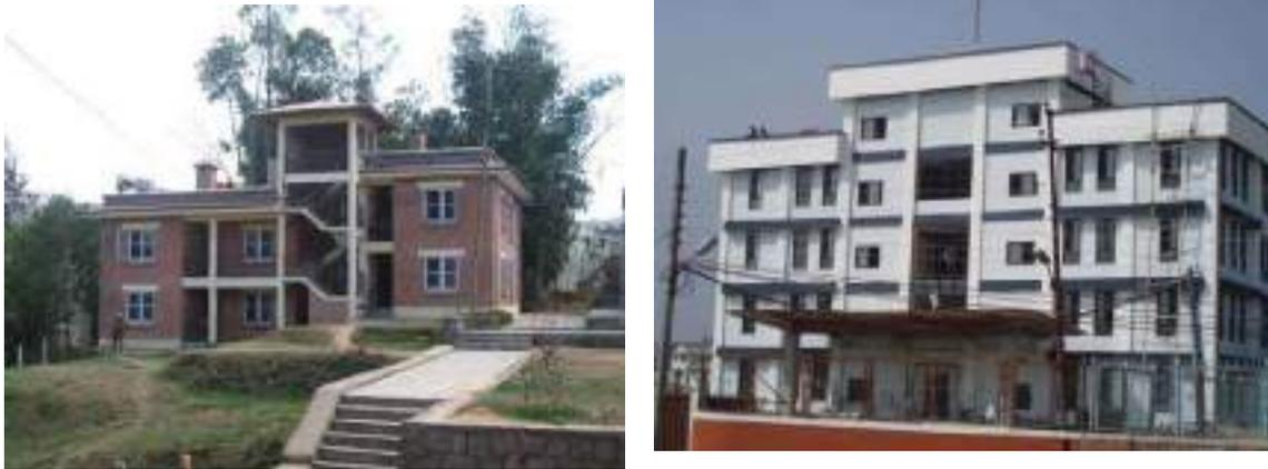
**Fig 1.4 Engineered Reinforced Concrete Moment Resisting Frame Buildings**
