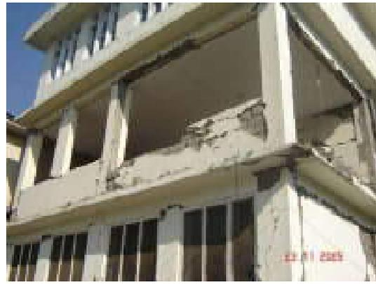
Cracks in column and beam at the base, spalling of concrete covers, buckling of steel bars, Large cracks in partitions and infill walls, failure of individual infill panels
