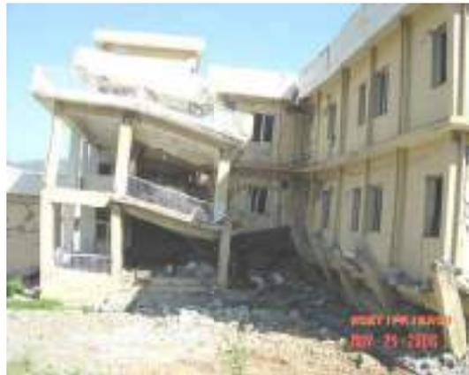
Photo 18: Earthquake damage due to soft story
