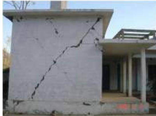
Photo 8: Diagonal cracking of solid wall
