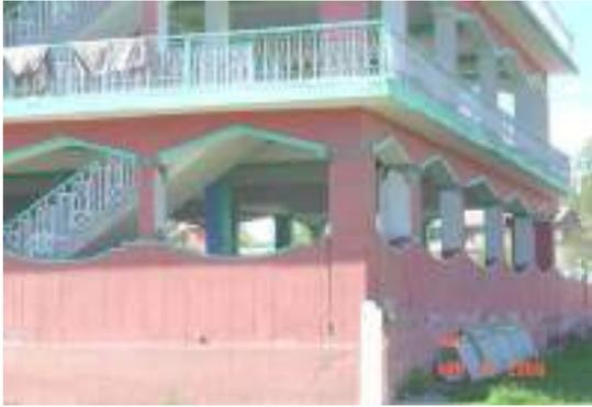
Photo 15: Slight-moderate damage
