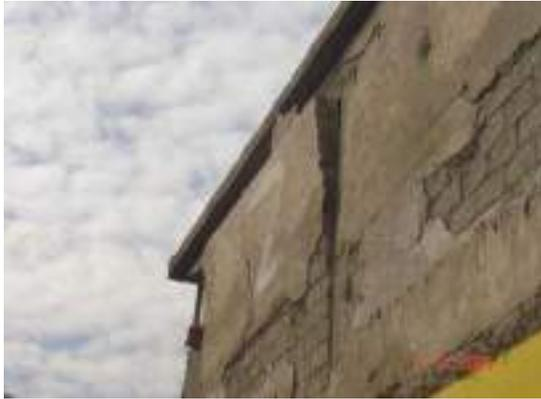
Photo 23: Moderate-Heavy Damage to Infill wall
