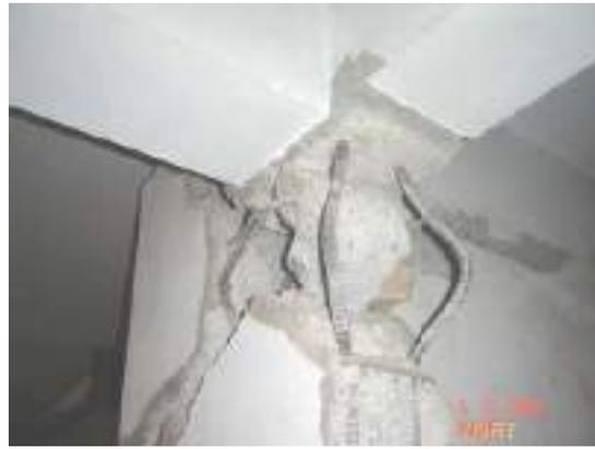
Photo 22: Buckling of column bars
