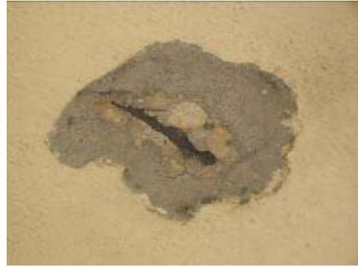
**Fig 2.9 (b) Rusting of Steel Bar**
