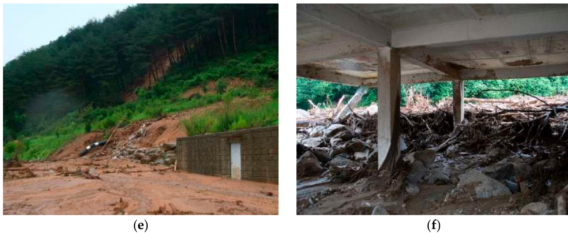
Figure 3. (a)–(e): observed landslides and (f) debris deposit.
