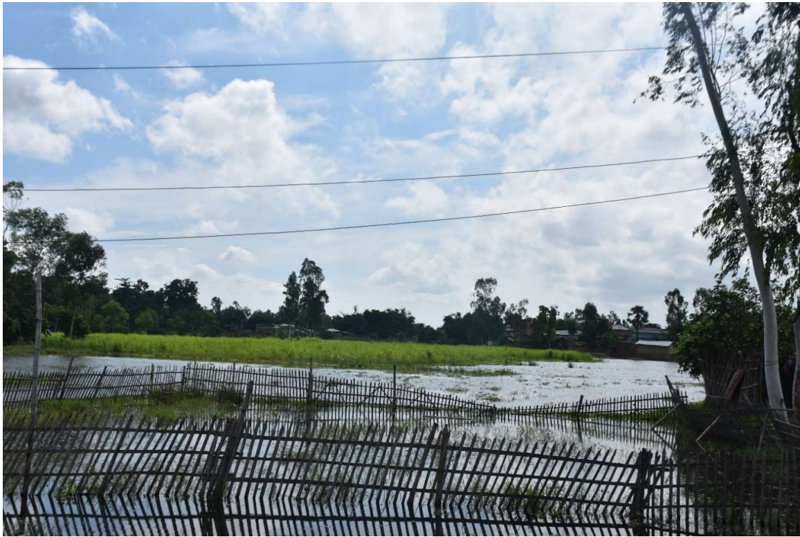
Inundation and local mitigation measures in Samsi Rural Municipality. Photo by Bhesh Parajuli on July 28, 2019.
