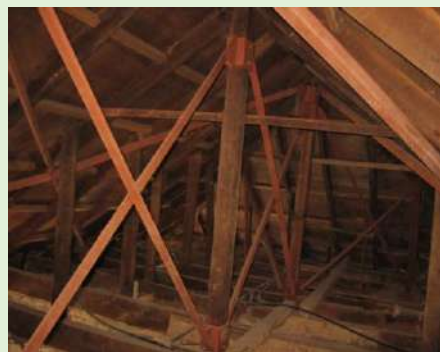
Steel bracing to roof
