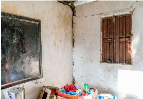
R.7.1 Low strength masonry : SMC
