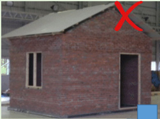
URM gable wall
