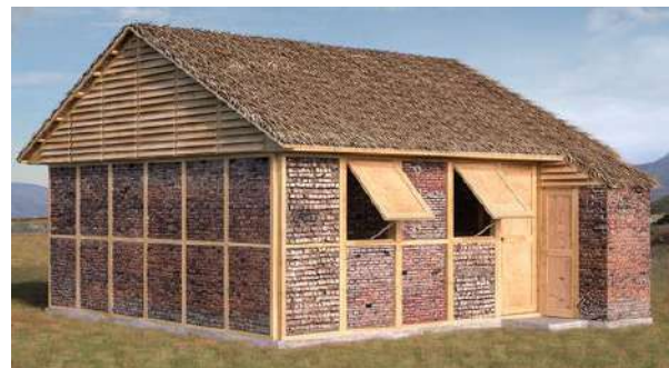
Use of timber planks at Gable part
