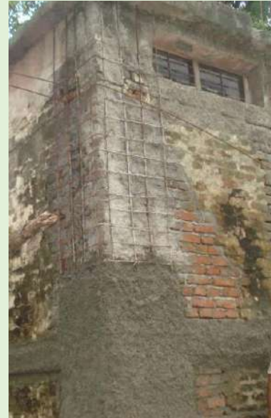
G I wire mesh anchored R C splint
