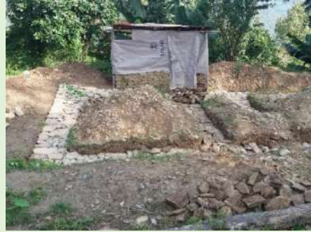
Insufficient foundation
