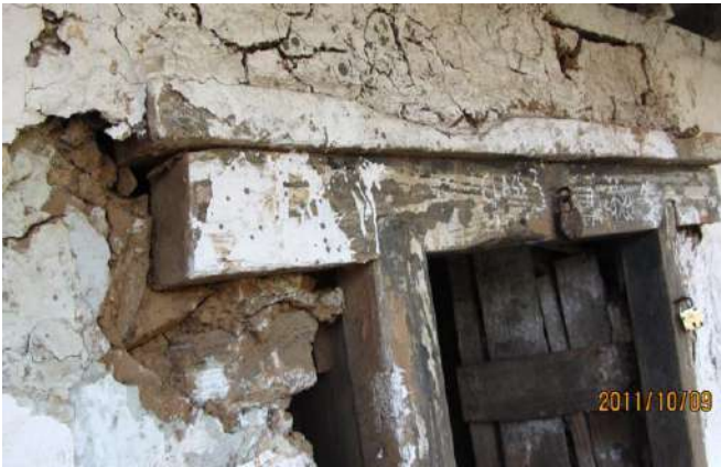
C.3.1 Low strength masonry : Stone Masonry in Mud mortar
