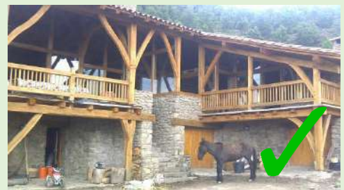
Wooden parapet with proper connection with floor joists
