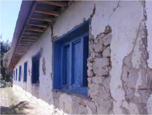
C2.1 Low strength masonry : Stone Masonry in Mud mortar
