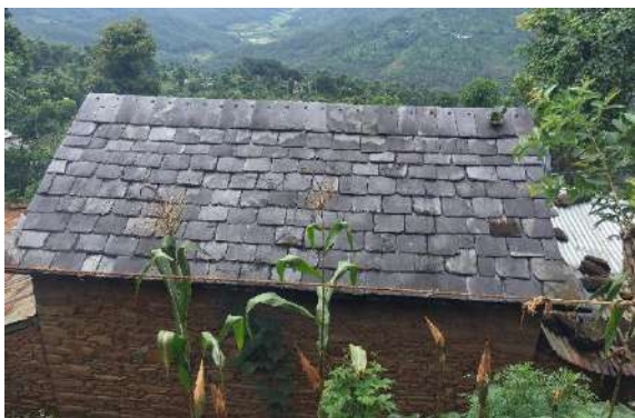
R.2.1 Slate stone roof
