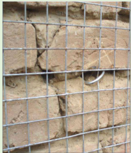
G I wire mesh anchored R C splint
