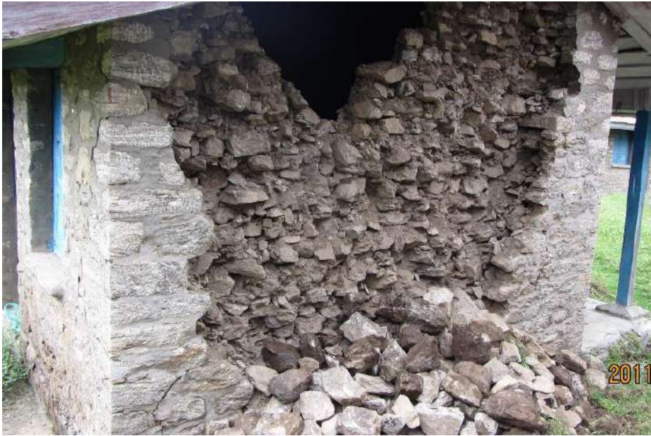
C.4.1 Low strength masonry : SMM
