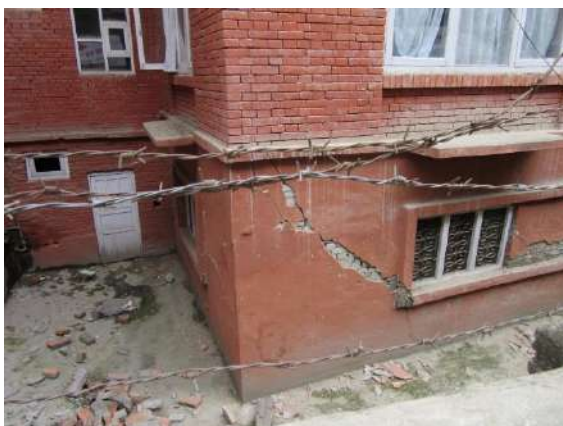
C2.3 Brick masonry in cement mortar
