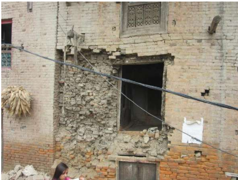
C.4.2 Low strength masonry : BMM
