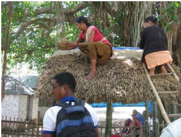
(Plastering with mud plaster)
