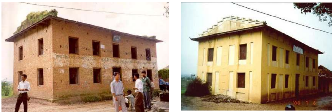
Fig. 6: Bhuaneshwori Lower Secondary School, Bhaktapur, the first retrofitted school by NSET, above pictures are of before and after retrofitting in 1997 (Source: NSET Archive)
