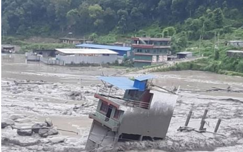
Flood has damaged as many as eleven houses in Melamchi Saturday night on July 31, 2021. The building of Radio Melamchi was also swept away in the flood. Photo: RSS
