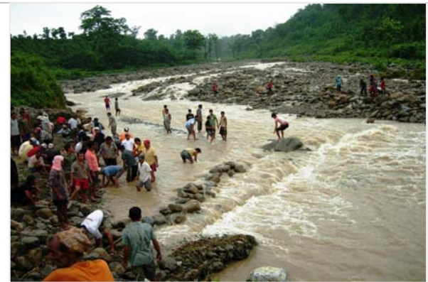
Farmers rebuilding the intake of irrigation channel after the cessation of rain. Photo: Tek Sapkota/Practical Action
